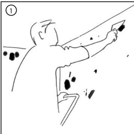
① Prepare the surface: fill in the holes. Remove the socket covers and switches.
